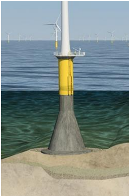
Figur 8. Gravitationsfundament. Illustration COWI
