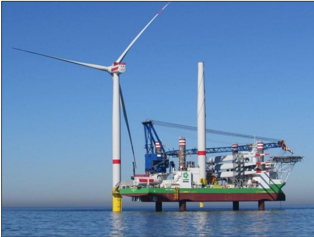
Figure 7. Installation of wind turbines using a jack-up vessel. Source: COWI
