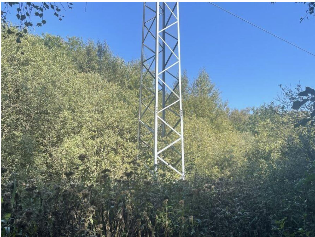
Figur 6: Mast 52. Foto: NIRAS, 8. september 2023.
