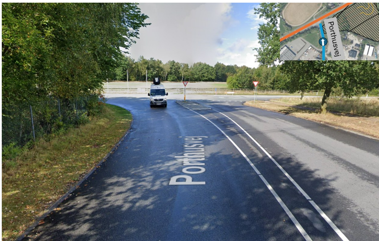
Figur 7-35. Porthusvej set mod nord (Google streetview, 2024)
