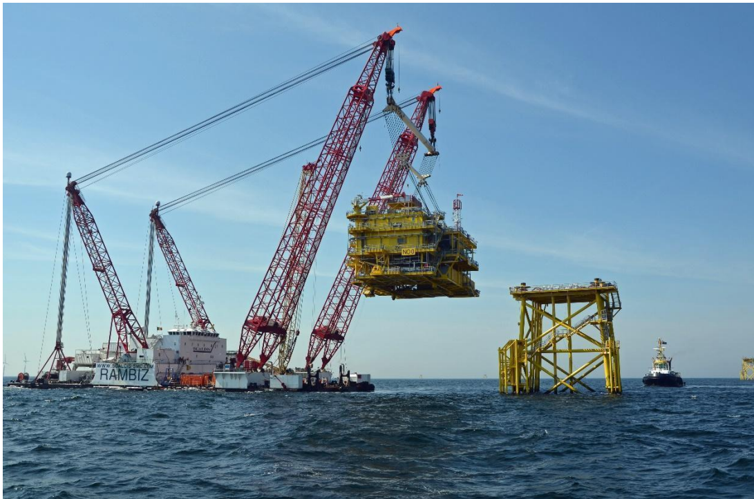
Figur 12: Offshore transformerstation under installation. Windpark Nordsee Ost havmøllepark (foto fra RWE resources)
