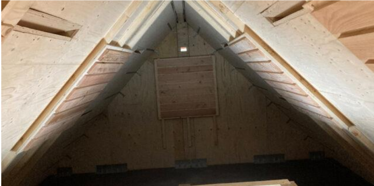
Figur 9. Indvendigt i bat barn https://www.fpcr.co.uk/new-bat-barn-within-area-of-natural-greenspace/
