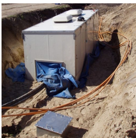
Figur 2-13 Muffecontainer
